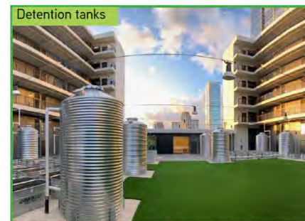
Detention tanks Store rainwater that can be reused for irrigation and indoor non-potable uses following plumbing codes Source: Artspace.org, "Olas Kailima Artspace Lofts", Honolulu.
